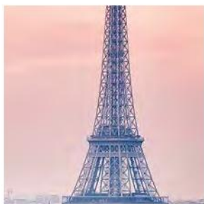
Torre Eiffel * 74987D97
